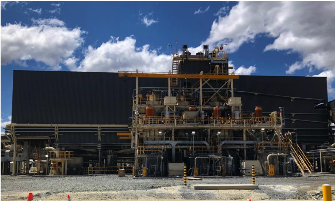
Figure 2 Flotation building during production this quarter.
