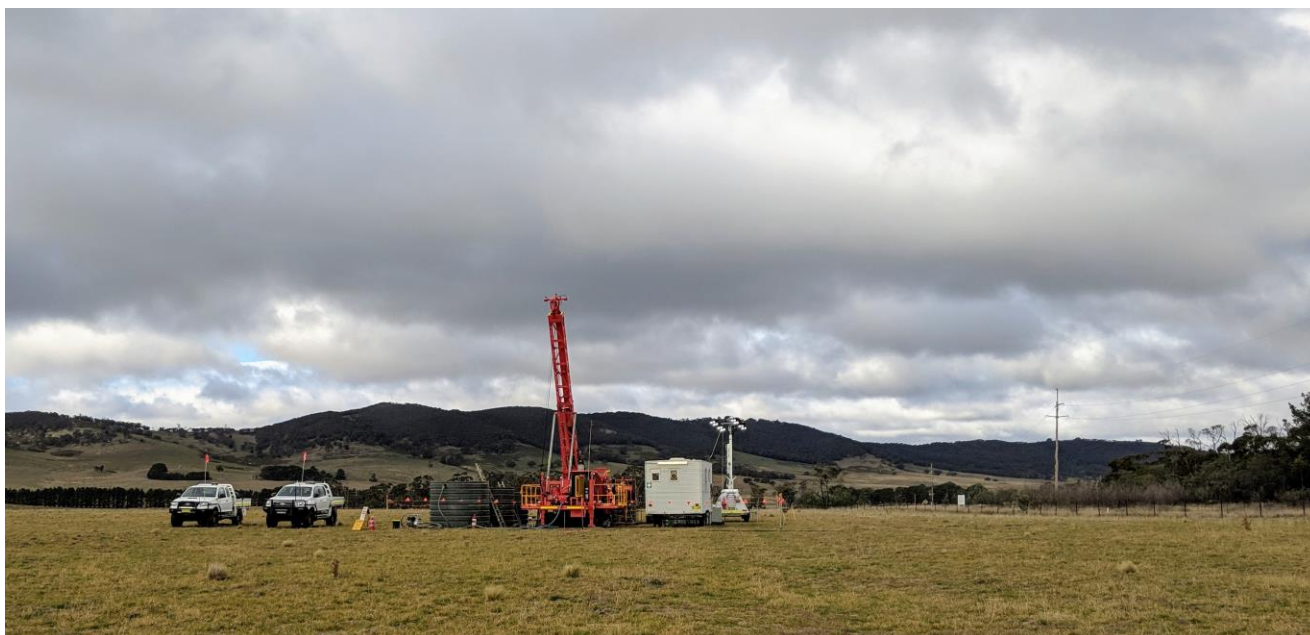
Figure 2: Drilling rig set up and drilling at the Murphy's IP target. Woodlawn processing plant 700m to the right.
