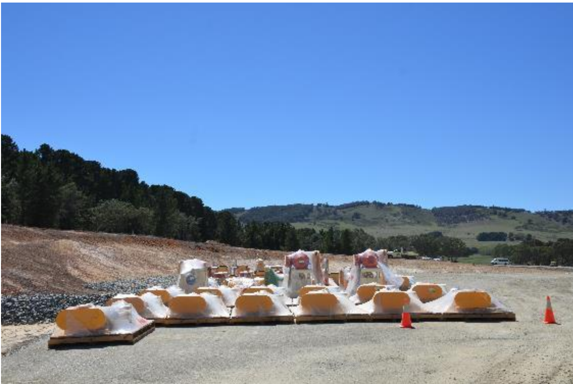
Figure 4: First process plant equipment deliveries.
