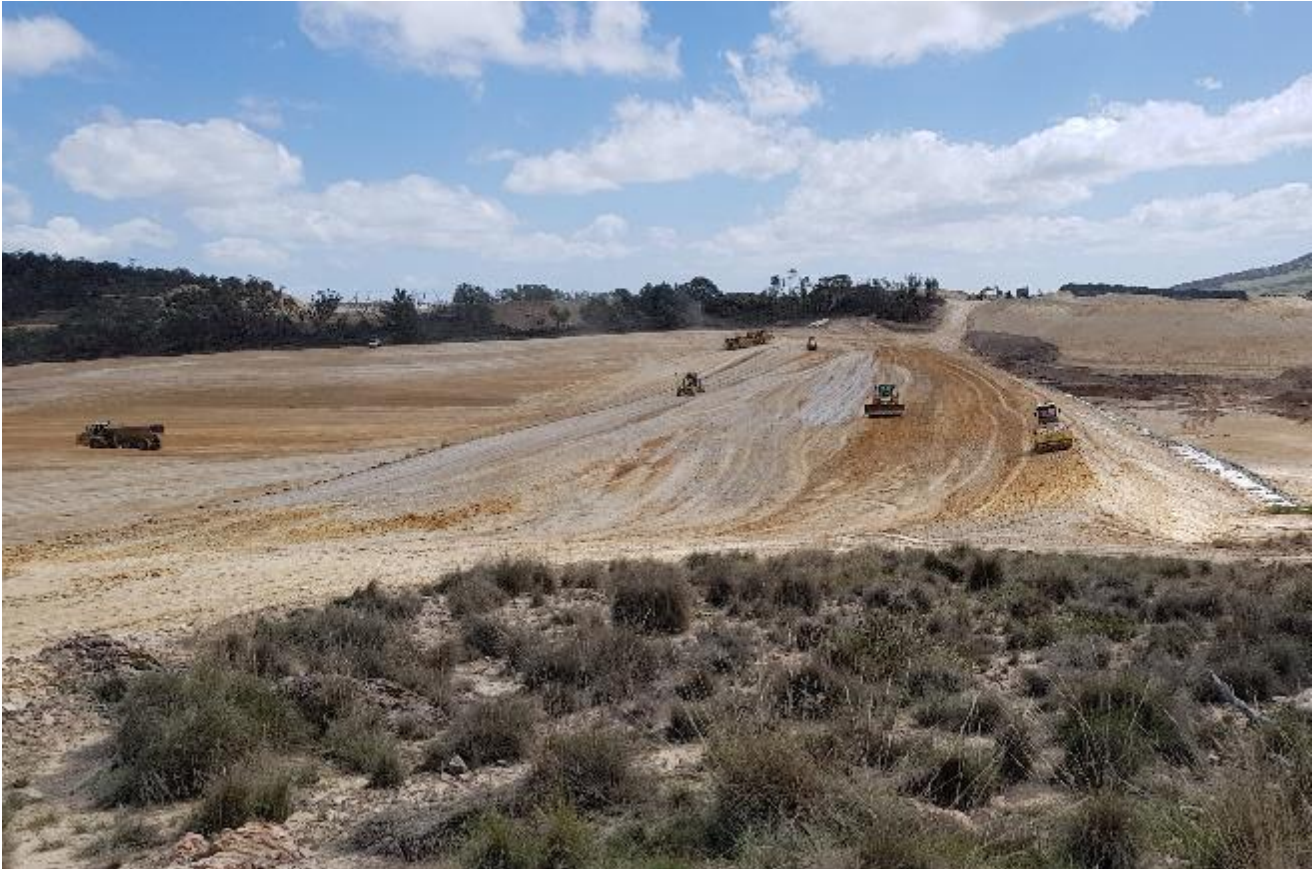
Figure 5: Tailings storage facility 4 construction.
