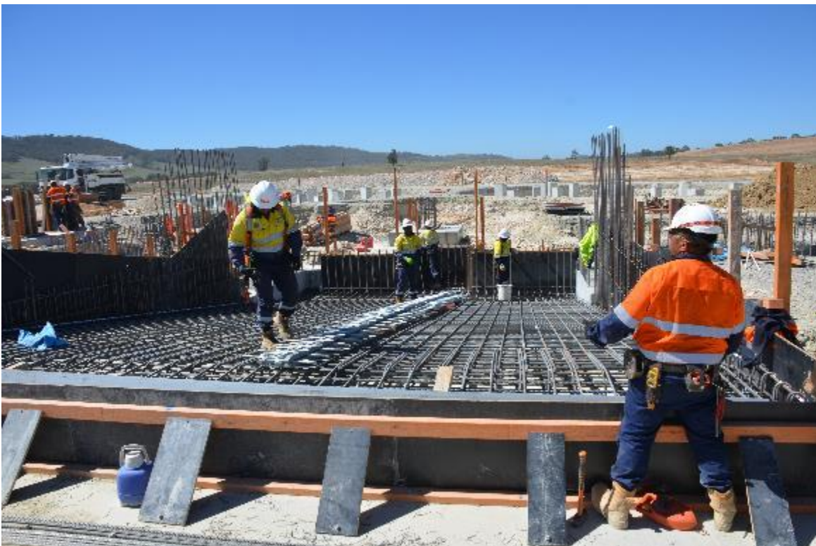
Figure 2: IsaMill foundations – reinforcing steel work.
