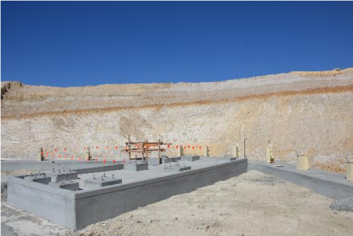
Figure 1: Primary crusher and ROM retaining wall foundations.
