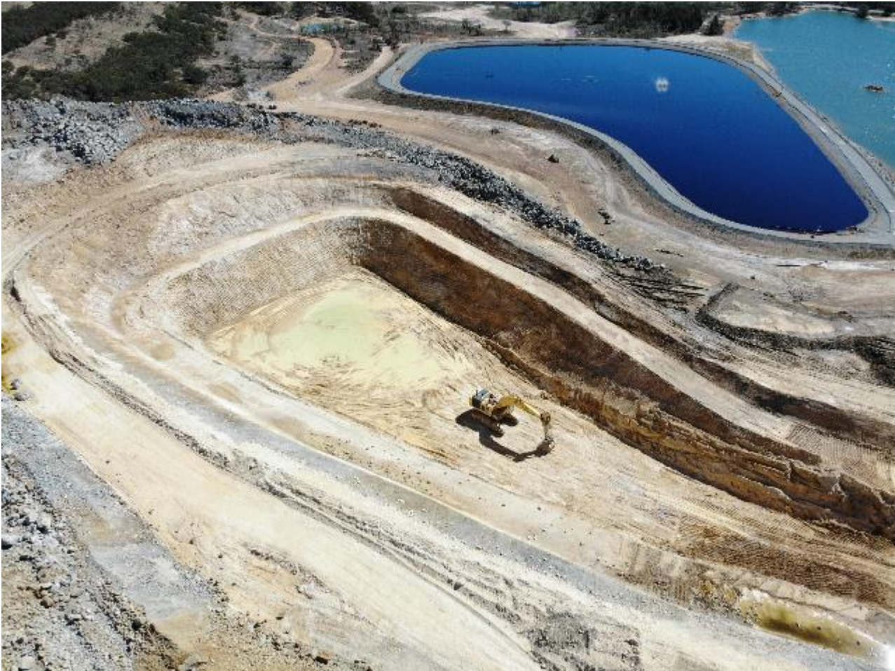
Figure 6: Box cut excavation – second bench.
