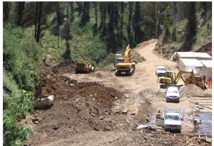
Pictured are site works at the A1 Gold Mine
