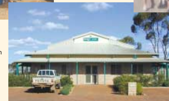
Heron Resources NL Exploration and Administration Office 21 Close Way, West Kalgoorlie
