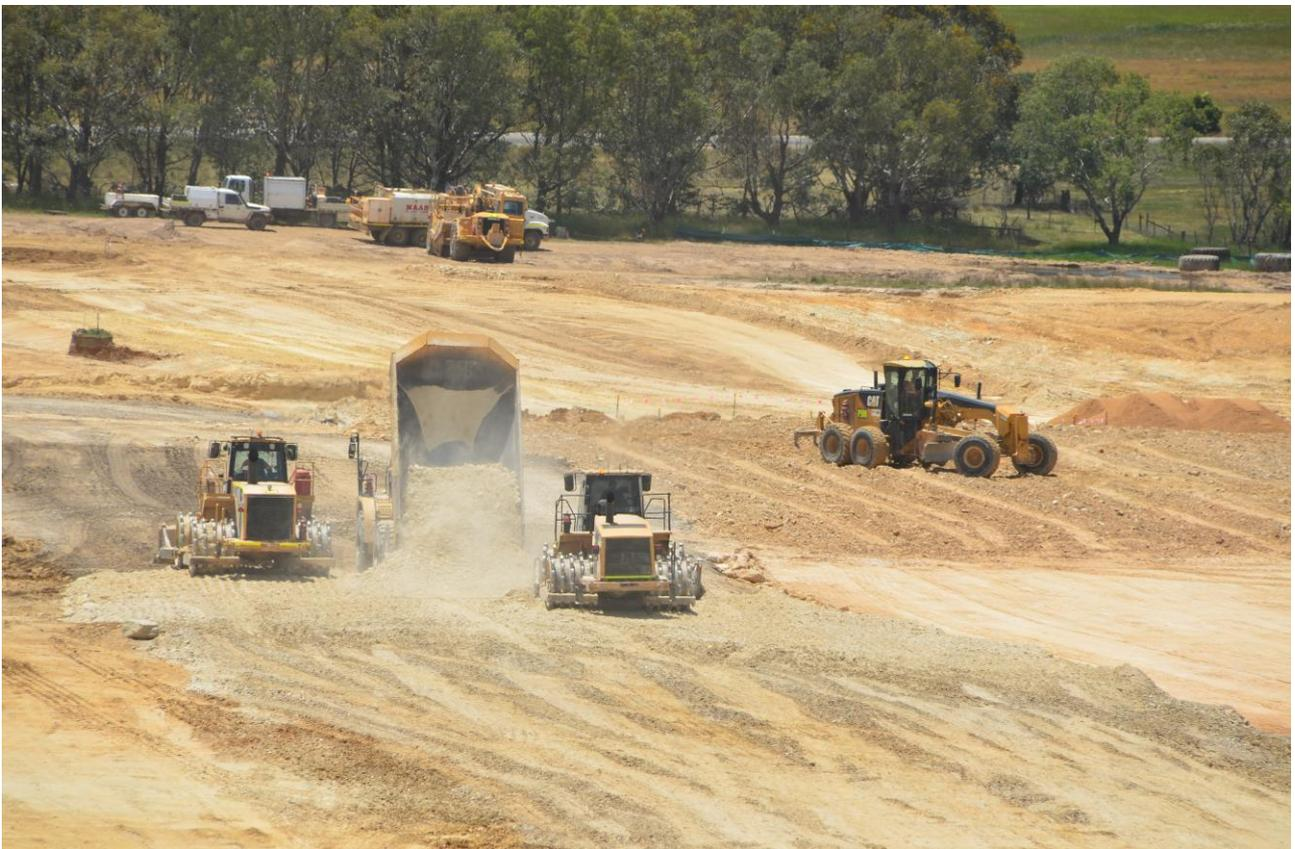
Figure 2: Process plant pad filling and compaction.
